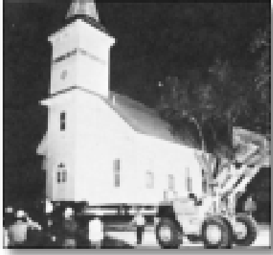
The 1889 Manatee Methodist Church being moved in December, 1975. Photograph courtesy of Manatee County Historical Commission
