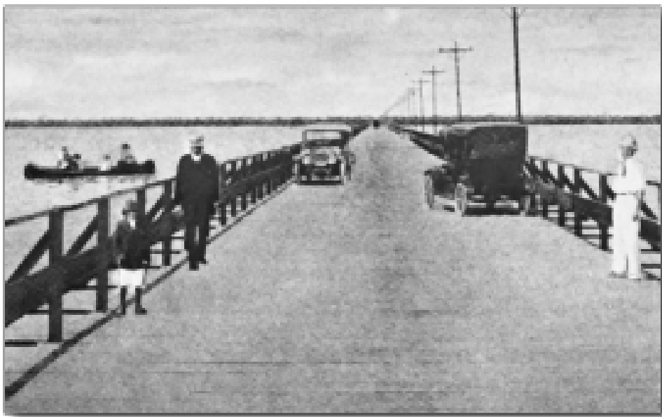
The bridge across Boca Ciega Bay from St. Petersburg to Pass-A-Grille, shown in a 1923 photograph.
